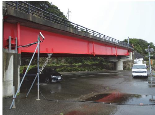
Figure 1. Exterior of the study bridge with three steel I-shaped girders.
