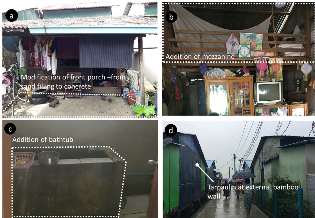
Figure 12: Changes in building elements (a) front porch, (b) mezzanine, (c) bathtub, (d) tarpaulin sheet
